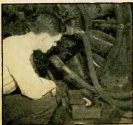
Fig. 2.—DON'T put them here! Strong fields from the cables may ruin the calibration.
